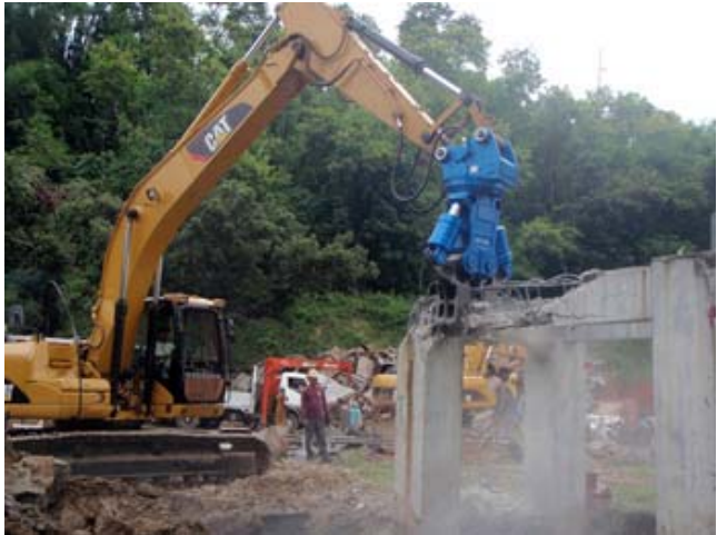
A Cat 320D equipped with an OKADA AIYON TSWK800V ARTS crusher is working on the site to break up the concrete structures.
